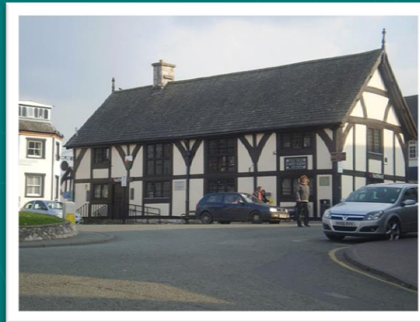
The Old Court House built in 1401
