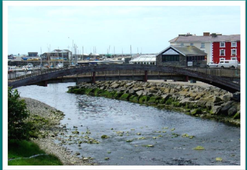
Footbridge over the Aeron
